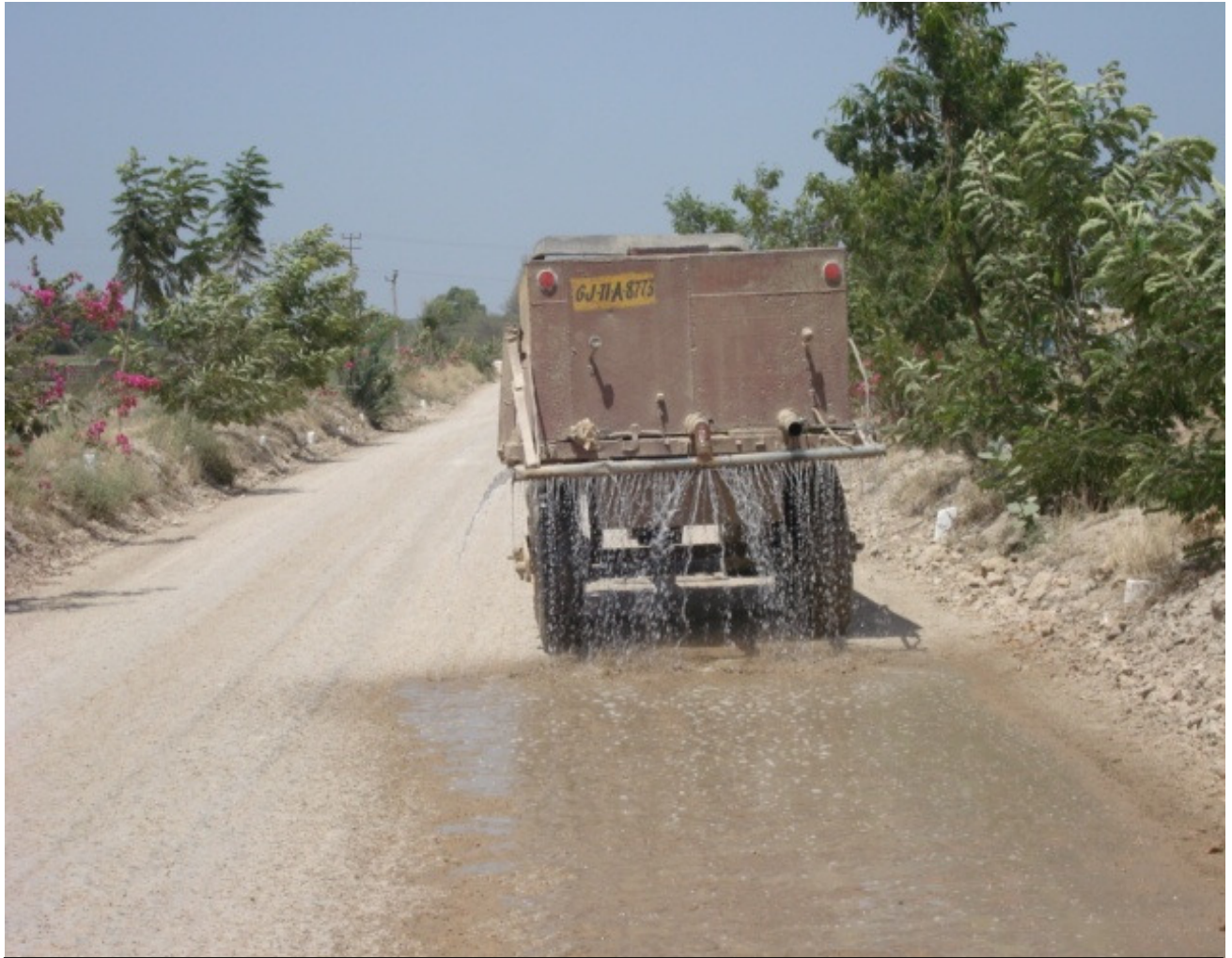
Regular Water Sprinkling is being done on haul roads in S No. 44 Mines
